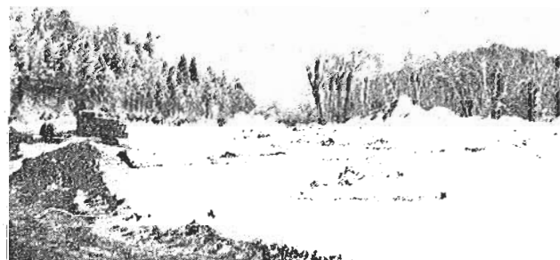
Piles of excavated material resulting from access road construction below the Teton Dam site. Wildlife officials wanted the road located above the canyon rim to prevent covering the shoreline habitat, destroying fish spawning gravels, and causing downstream siltation in the river.
