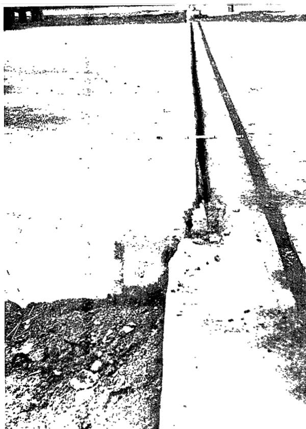
Separation of roadway and bridge abutment.
