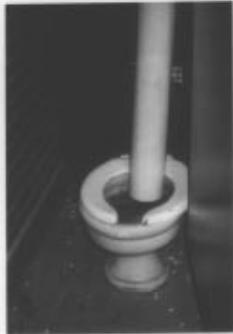
**Toilet Used to Redirect Sewage From Broken Pipe in Wall**
