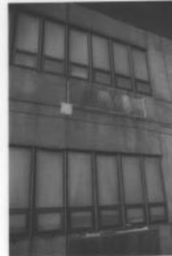
**Coming Apart at the Seams: Cracked Demountable Classrooms Held in Place by Steel Plate; Wall Crumbling Under Windows**
